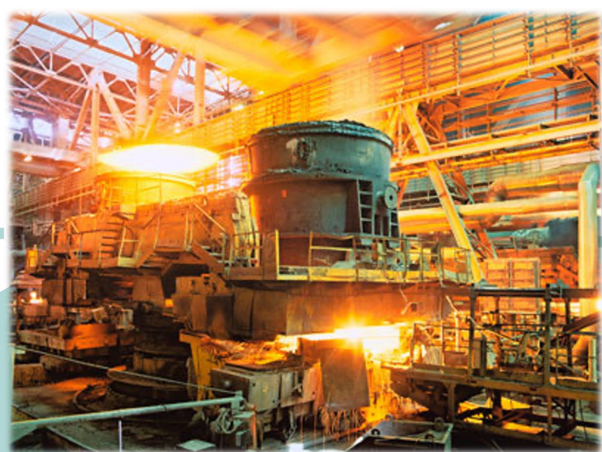
Zhezkazgan copper-smelting plant (出典: AZERNEWS)
